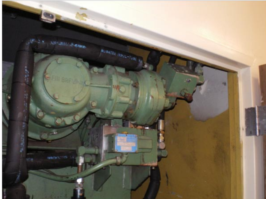
Figure 7: Drive Unit #1 small space available
